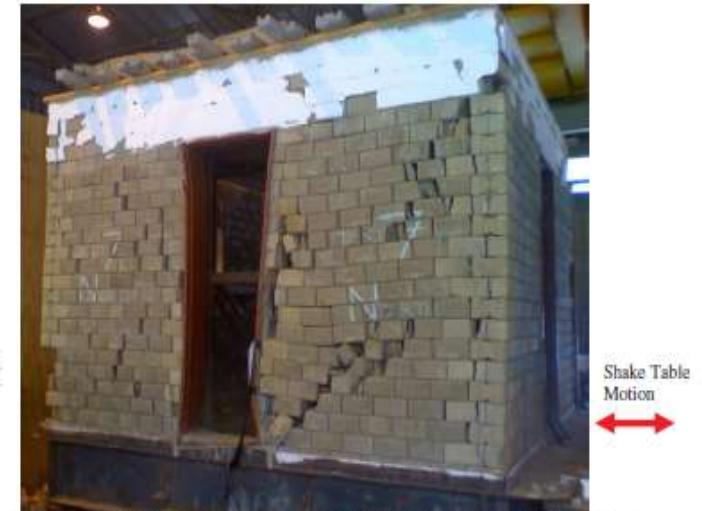
Figure 13: Damaged test structure showing the North wall after the base is subjected to a 22 mm, harmonic 3 Hz motion for 15 seconds.
