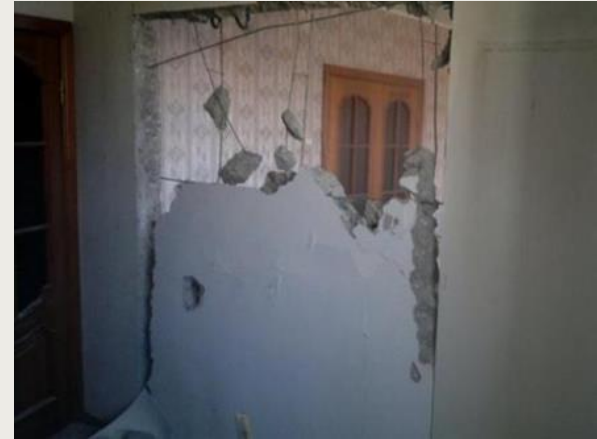
Partial removal of façade panel to utilise the balcony and increase usable space and increasing of a door opening /a new door (right)
