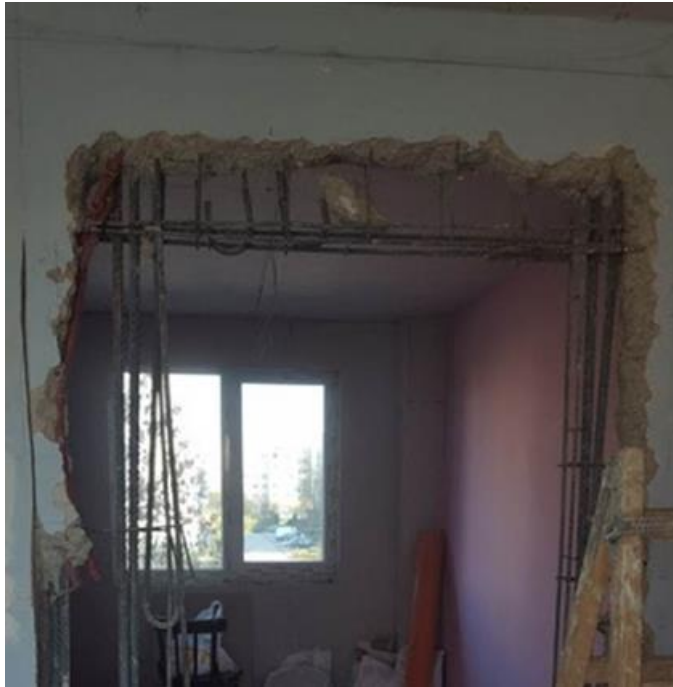
Increasing the size of a door opening
