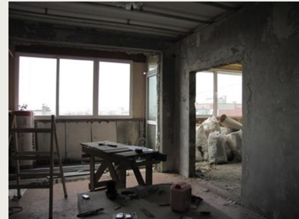
Partial removal of façade panel to utilise the balcony and increase usable space and increasing of a door opening /a new door (right)
