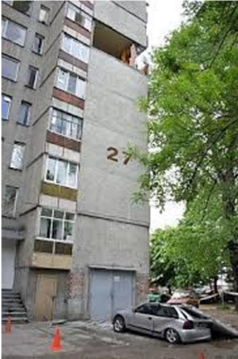
Façade panel fallen onto a parked car in Stara Zagora (corroded connections)
